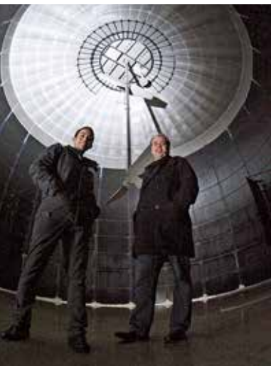
Michael Martin and Mats Eklund in a biogas reactor that is not yet in operation.
